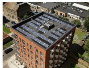
Figure 3.21 - PV installation on building with flats
