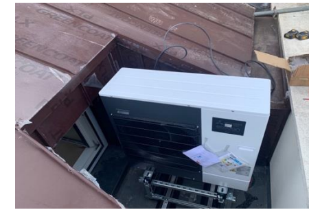
Figure 3.13 - Roof mounted air source heat pump
