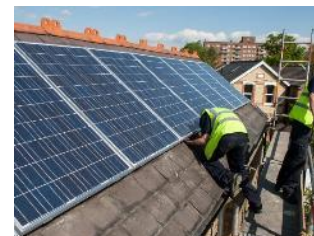
Figure 3.19 - PV installation over the tiles
