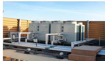
Figure 3.14 - A centralised heat pump system on the roof of a building
