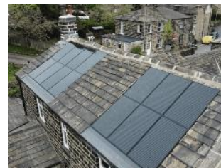
Figure 3.18 - PV installation as tile replacement
