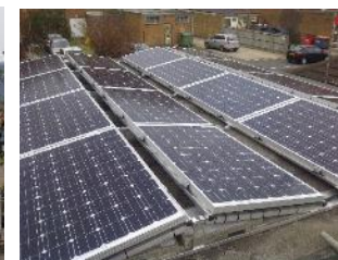
Figure 3.22 - PV installation over tiles
