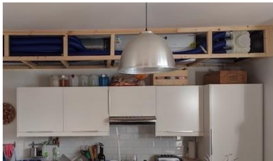
Figure 3.11 - MVHR units can be retrofitted into ceiling voids or wall mounted (© Will South) Ductwork has to be routed to every room. A qualified installer and/or an MVHR manufacturer/supplier will be required to calculate the fresh air required and to design the ventilation system.
