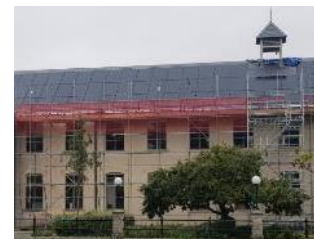
Figure 3.22 - PV installation over tiles
