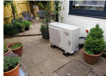
Figure 3.12 - Front/ Rear garden – ground mounted air source heat pump
