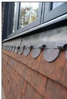
1 SCALLOPED LEAD FLASHING DETAIL
