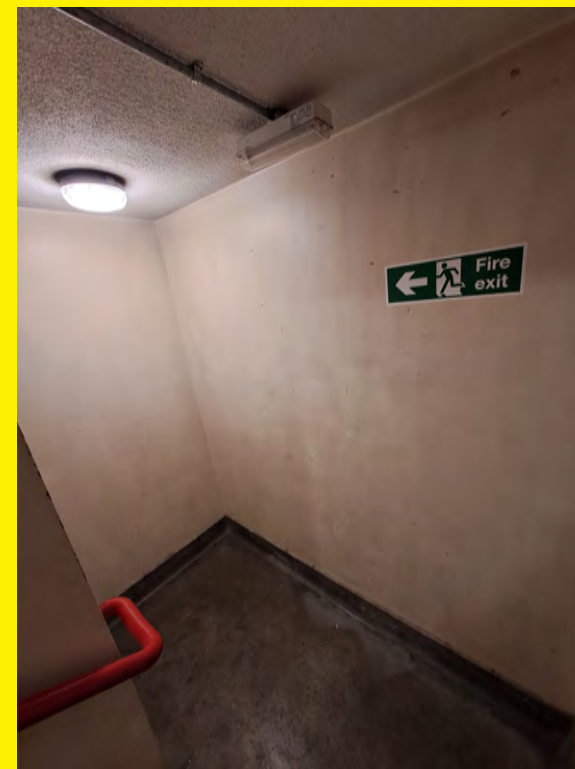
Stairwell emergency lighting at 40 Hampstead Road.
