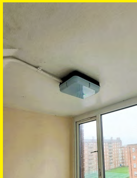
Internal and external emergency lighting at Castle Court.
