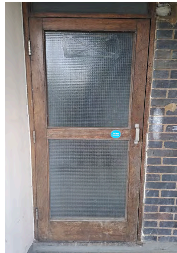
Internal staircase fire door at Barrington Court.
