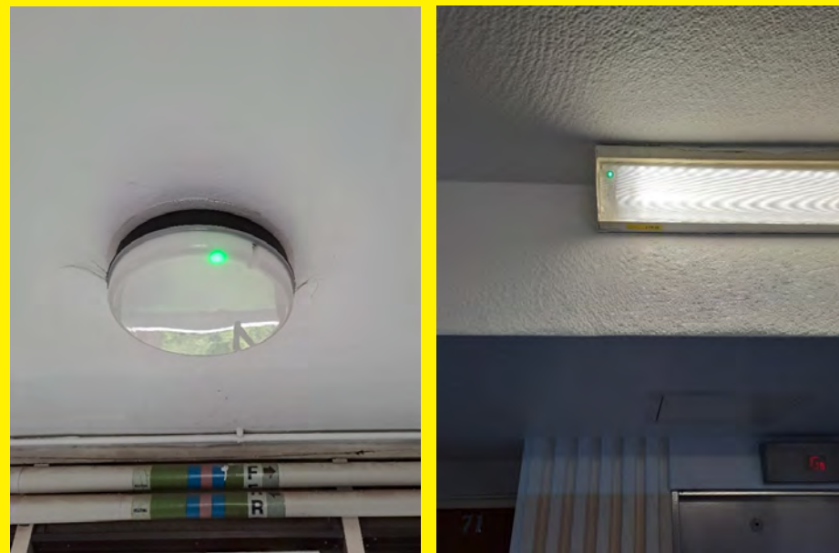
Various Emergency Lighting at Blashford Tower.
