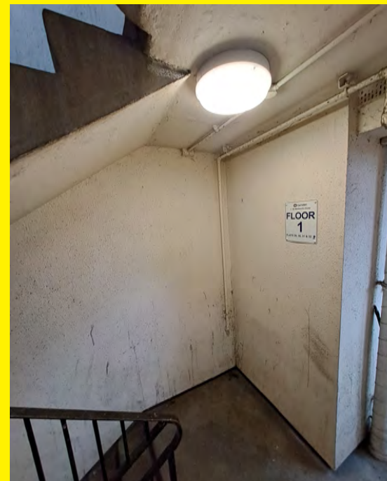
Emergency lighting in the stairwell at Mackworth House.
