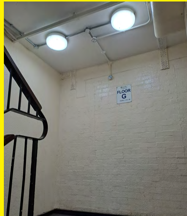
Emergency lighting in the stairwell at Hawkshead.
