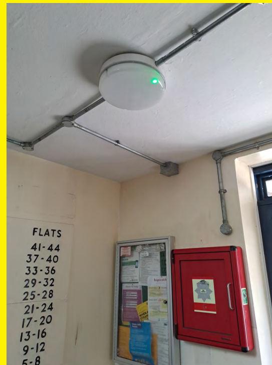
Emergency lighting and Secure Information Box at Swallowfield.
