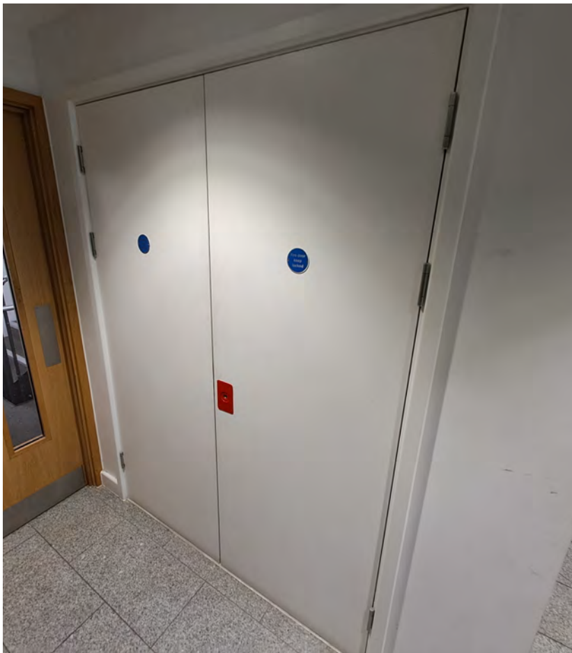
Service Riser Cupboard Fire Door at Winchester Apartments.
