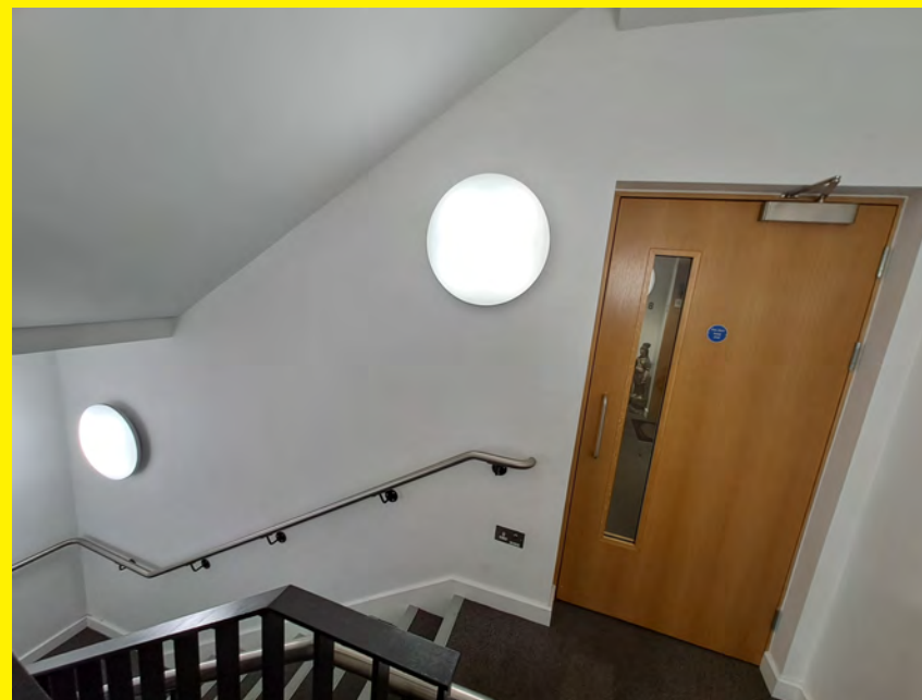
Stairwell emergency lighting Winchester Apartments.
