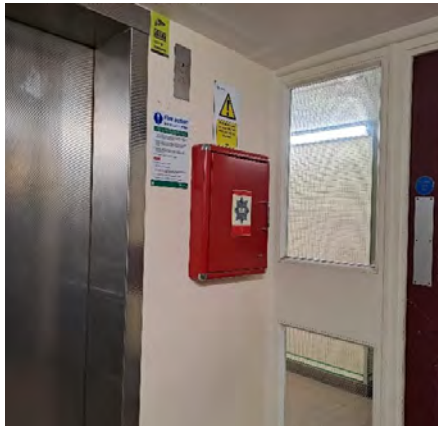
Secure Information Box at Bray Tower.
