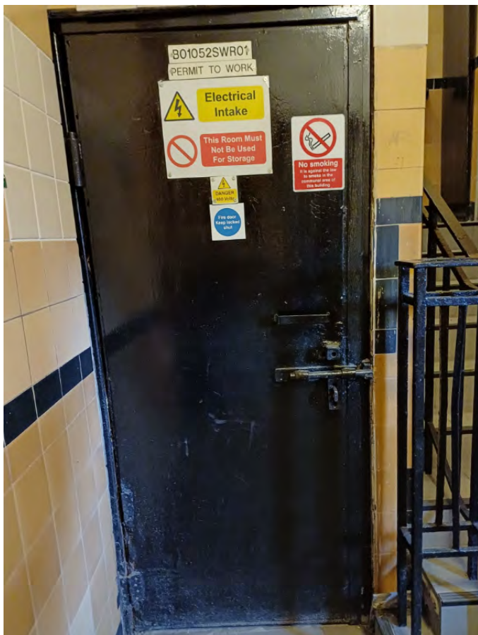
Electrical intake cupboard fire door at 1-24 Tottenham
