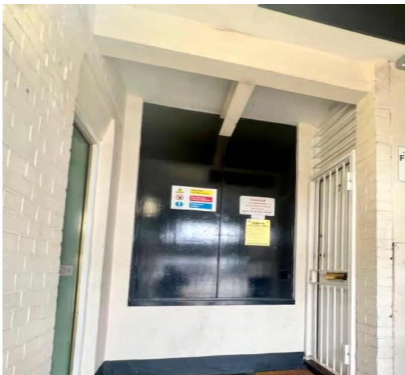
Electrical cupboard Fire door at Cavendish Mansions.
