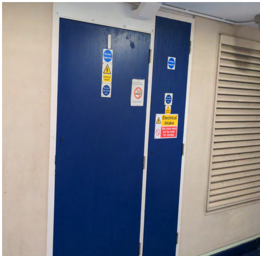
Electrical Intake Cupboard fire door at Lulworth Tower.
